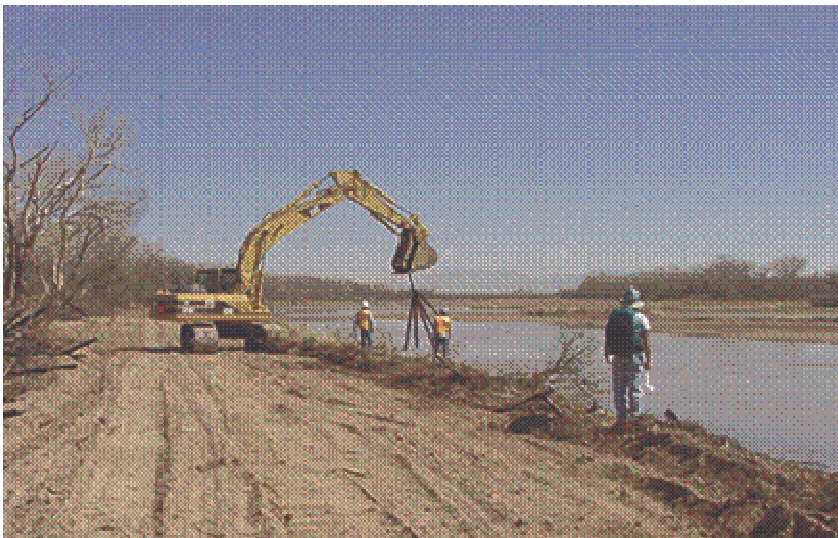
Removing a jetty jack from the riverbank.
