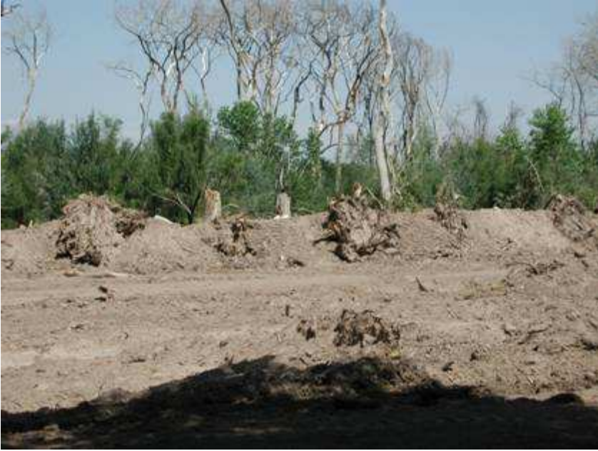
Cottonwood root wads used to fortify the levee. Burned cottonwood trees are in the background.
