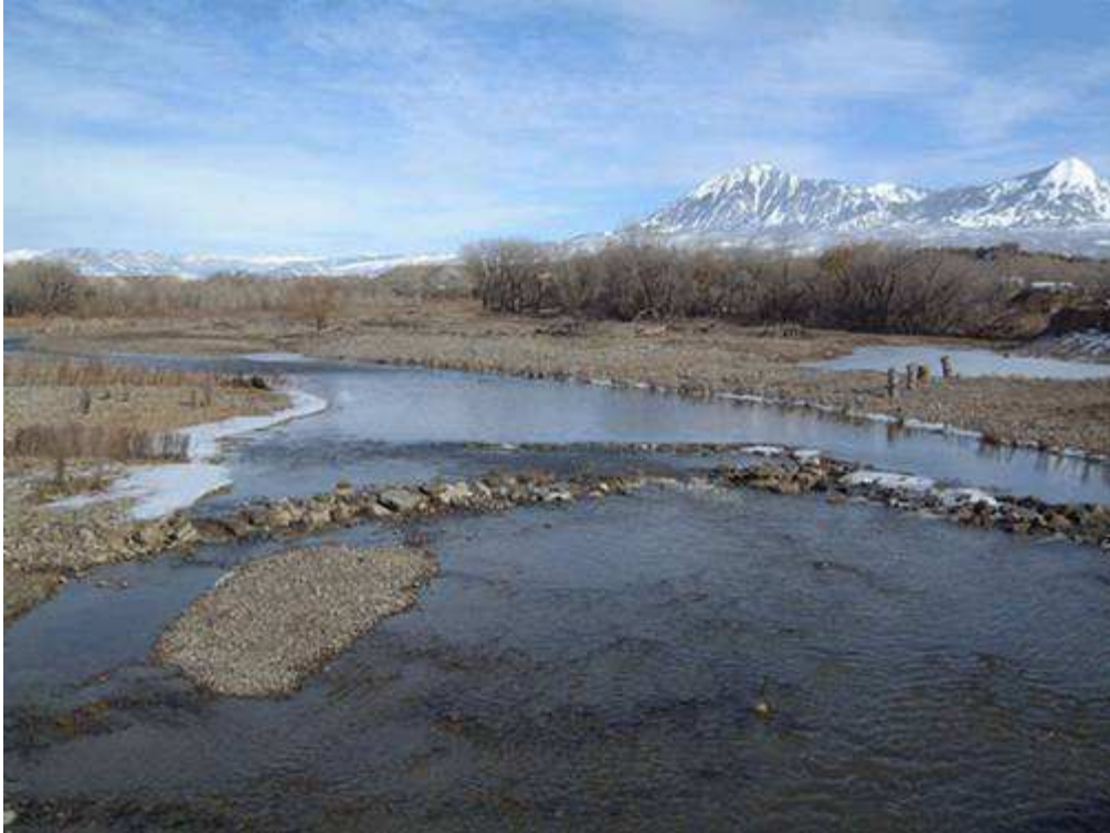
New weir constructed as part of the Hotchkiss Demonstration Project
