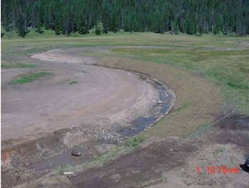
Red River restoration reach under construction
