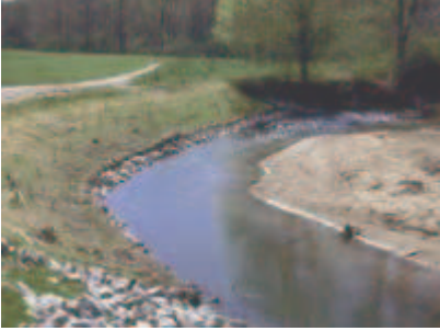
Immediately after restoration of Cinnamon Creek, April 2001 (photo courtesy of Northern Virginia Soil and Water Conservation District)
