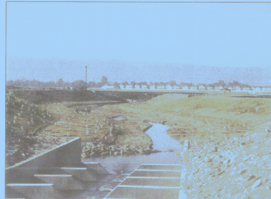
Photo Station 5: from northeast end viewing southwest (Jan. '04)
