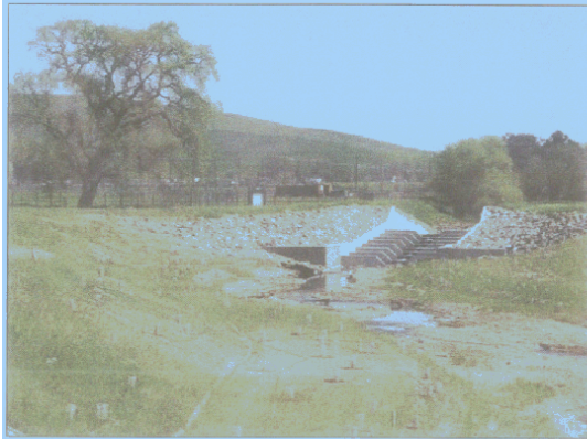
Photo Station 4: from Vulcan Bridge viewing east (Mar '04)
